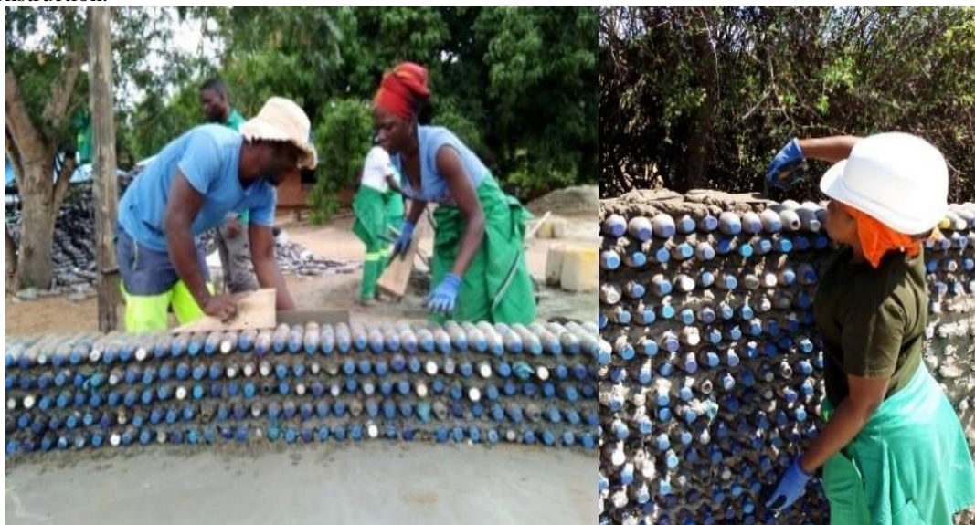
Figure 02 and 03: Placement of plastic bottles to form the structural walls during the construction process. Source: Yopipila Project Archive (2024)
