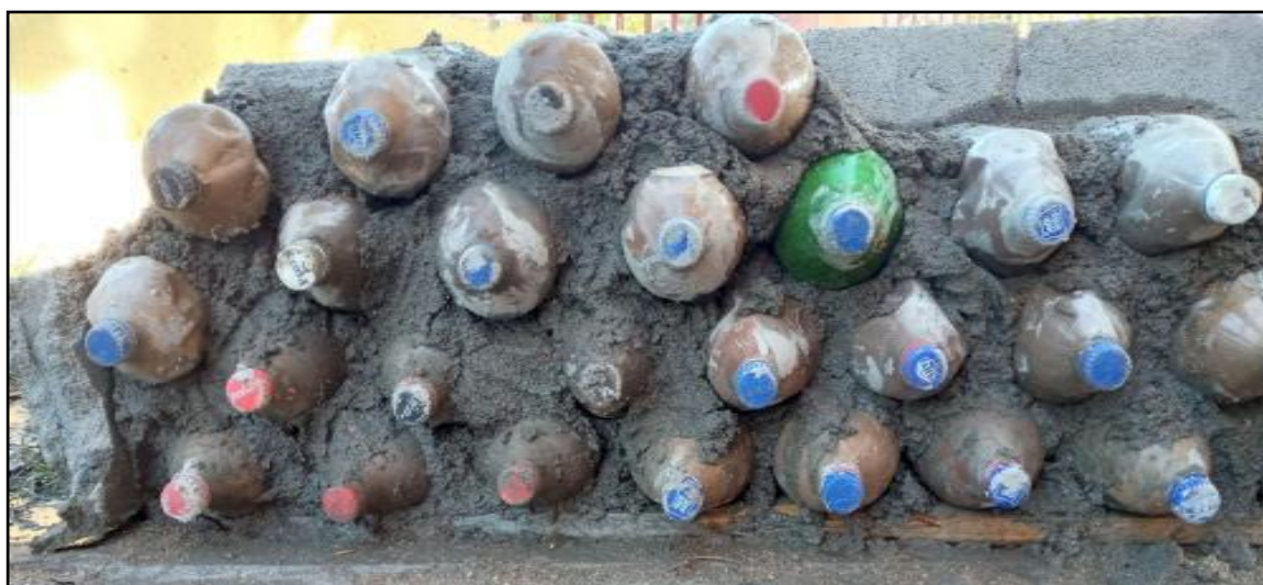
Figure 04: Prototype of a wall made of plastic bottles filled with wet soil Source: By Author (2024)
