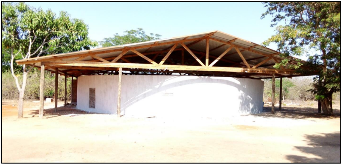
Figure 05: Final state of one of the plastic bottles houses Source: Yopipila Project Archive (2024)
